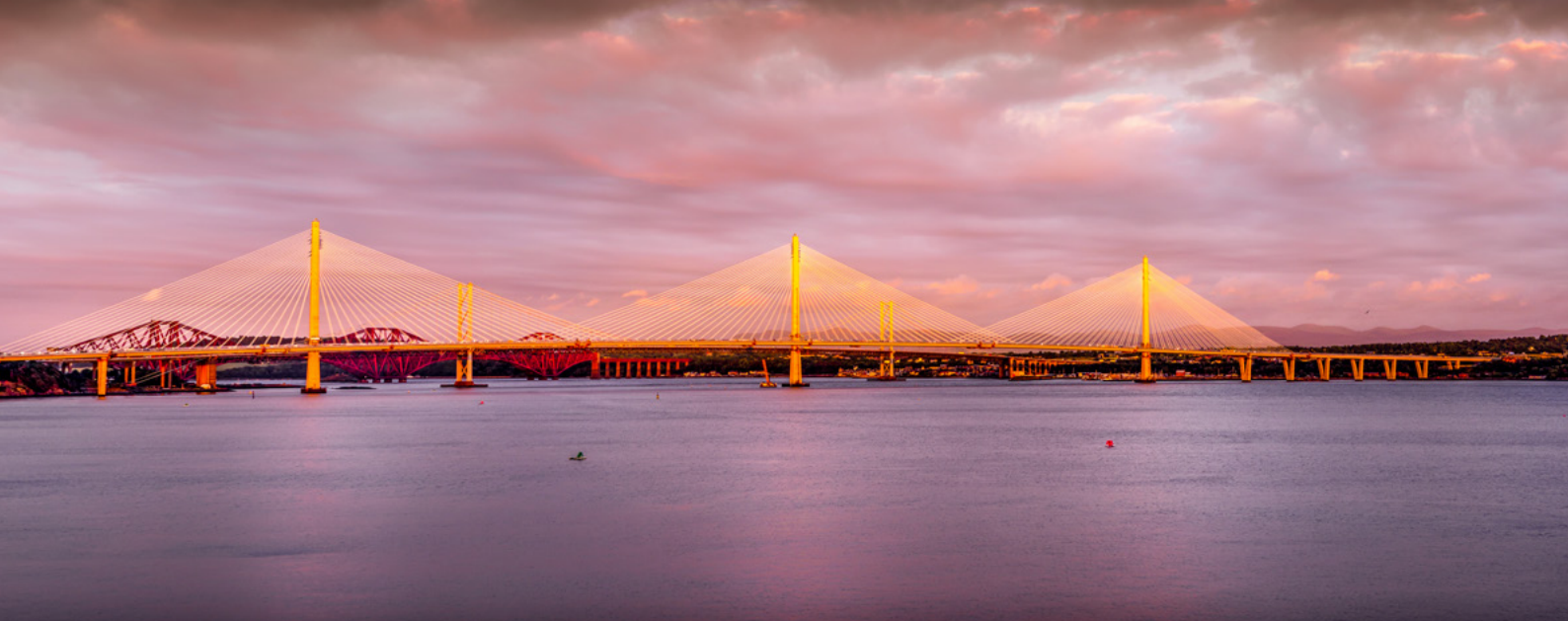
Queensferry Crossing, Firth of Forth, Scotland
